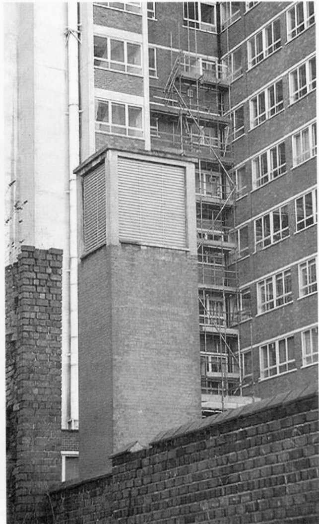
Ventilation shaft for the Anchor deep level trunk exchange in Birmingham - Photo by Sebastian Ballard
